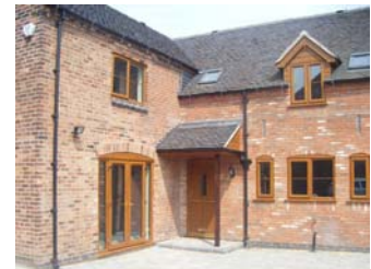
New Courtyard Entrance
