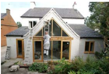
New Rear Extension
