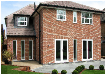
West Bridgford: New Rear Extension
