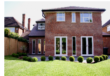
West Bridgford: New Rear Extension
